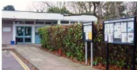
Thames Ditton Centre for the Community
